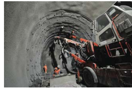
Baustelle Sigirino Photos Alp Transit San GottardoSA
